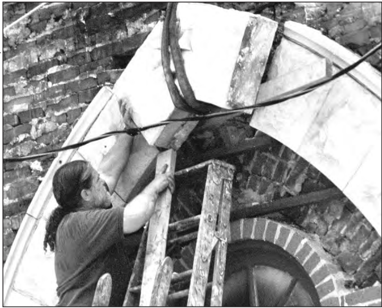
Tim Harmon, of Tim and Billy's Salvage of Indianapolis, works to save the original arch from Holy Cross Central School before the school is demolished. The arch is expected to be used for the entrance of the pre-kindergarten building.
